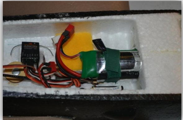
On my older T-28, I added a Velcro strap to help secure the battery in place. I've never had an issue with this set-up.
