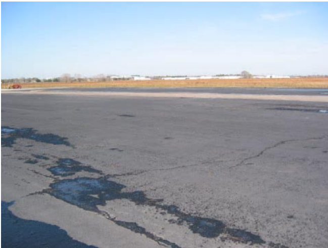
View looking west from Tx impound
